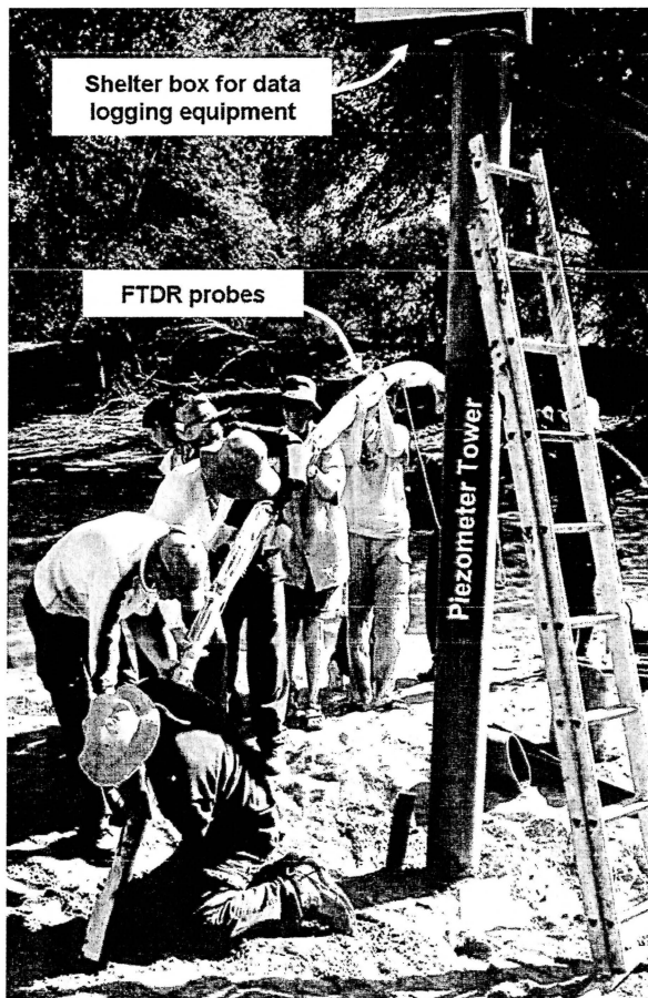
Figure 4. Installation of the FTDR probes in a slanted borehole beneath the stream channel.
